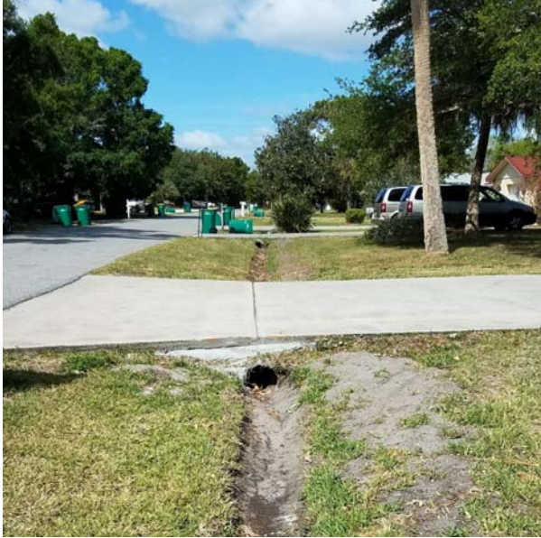
Local street-side swales correctly cleared of debris
