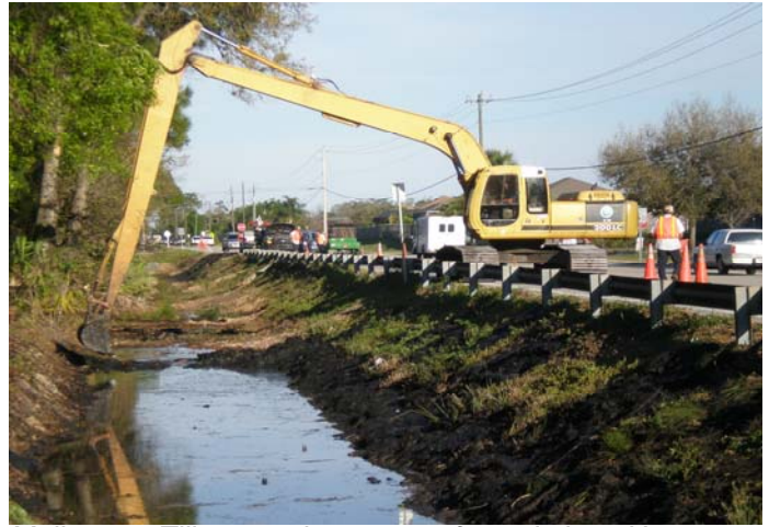
Melbourne-Tillman maintenance of canal along Henry Avenue
